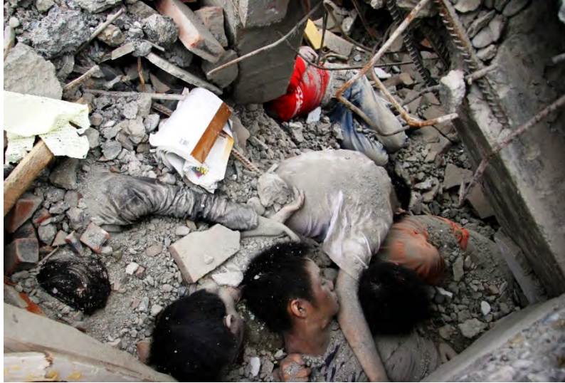
Middle school after earthquake. 3
